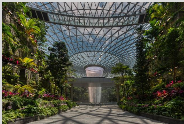
l. ) Jewel Changi Airport (Safdie Architects)
